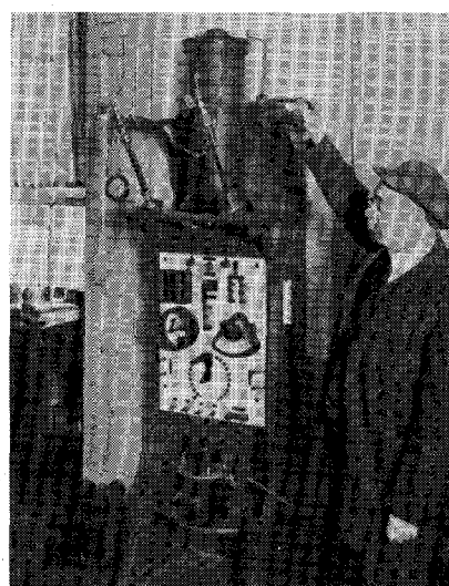
Fig. 4. D'Arsonval adjusting the spark gap of his improved high-frequency generator [88].
